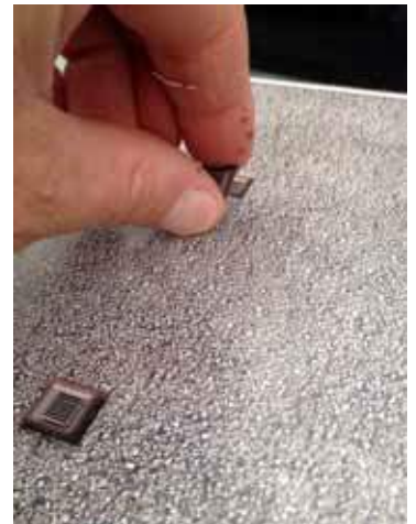
Add roof vents with spacers
