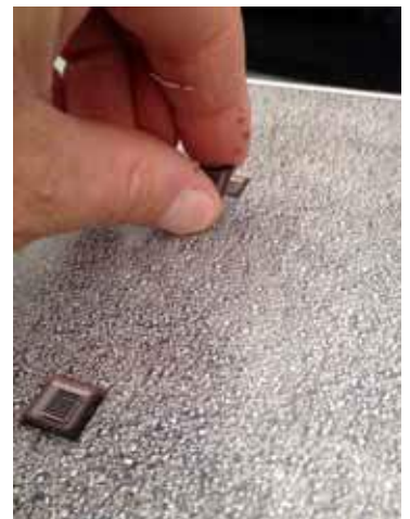
Add roof vents with spacers
