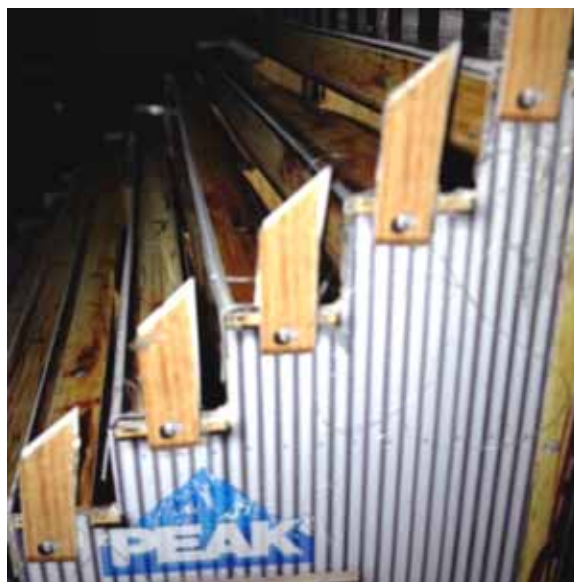
Figure 19 - Attach the handrail supports.
