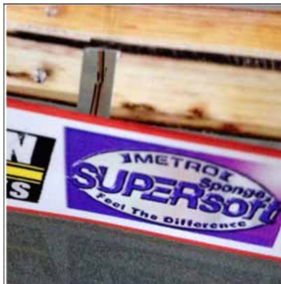
Figure 18 - Notch the lowermost bleacher.
