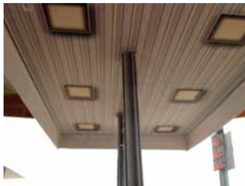
Under canopy detail view
