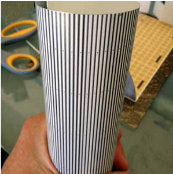
Figure 9 - Roll the roof material to pre-form it.
