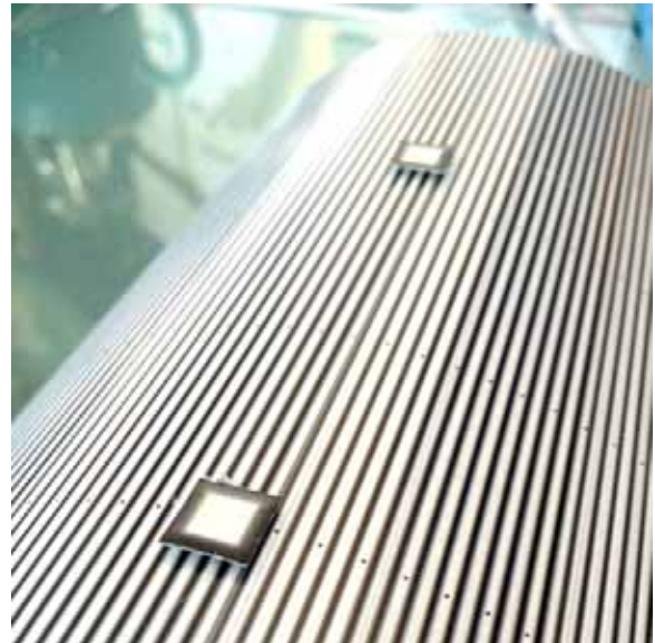
Figure 14 - Position and attach the vent pieces to the roof.
