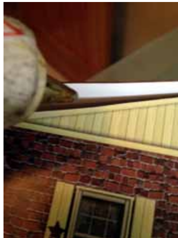
Finish attaching roof
