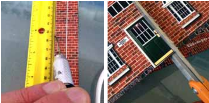
Figures 4-A, 4-B – Score the hinge side and cut the swing side of the doors to open.
