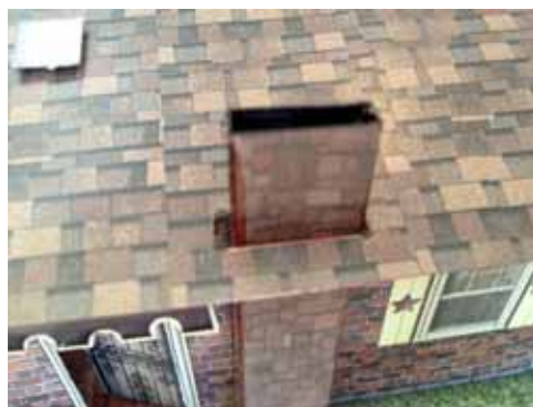
Roof and chimney detail
