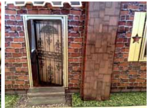
Side entrance detail
