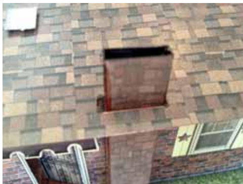
Roof and chimney detail
