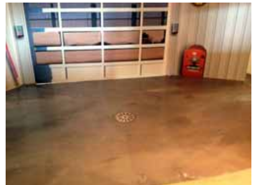
Interior detail view
