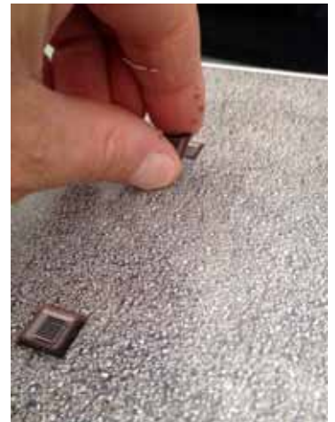
Add roof vents with spacers
