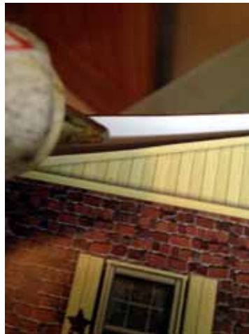
Finish attaching roof
