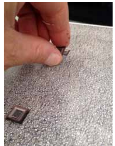
Add roof vents with spacers
