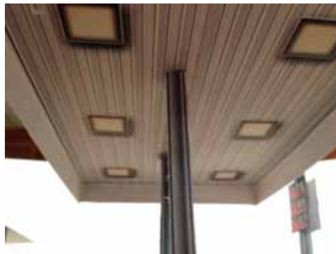
Under canopy detail view
