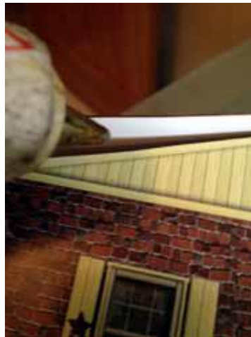
Finish attaching roof
