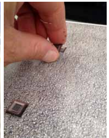
Add roof vents with spacers
