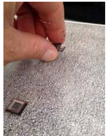
Add roof vents with spacers
