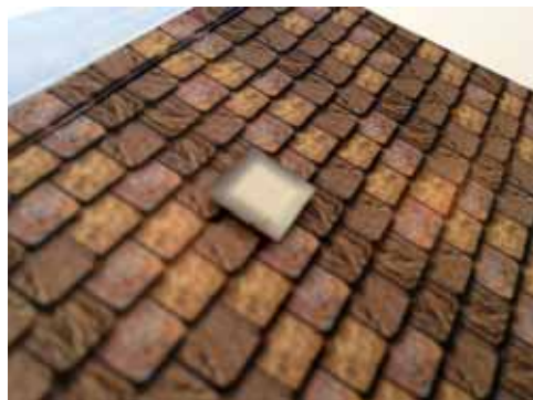
Roof top-down view
